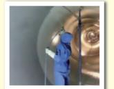
Depending on the circumstances, AB-COR® 950 SW, AB-COR® 950 SW-H, AB-COR® 955 SW and AB-COR® 955 SW-H can be used as a single or multi coat system, easily applied with a suitable one-component airless sprayer.
